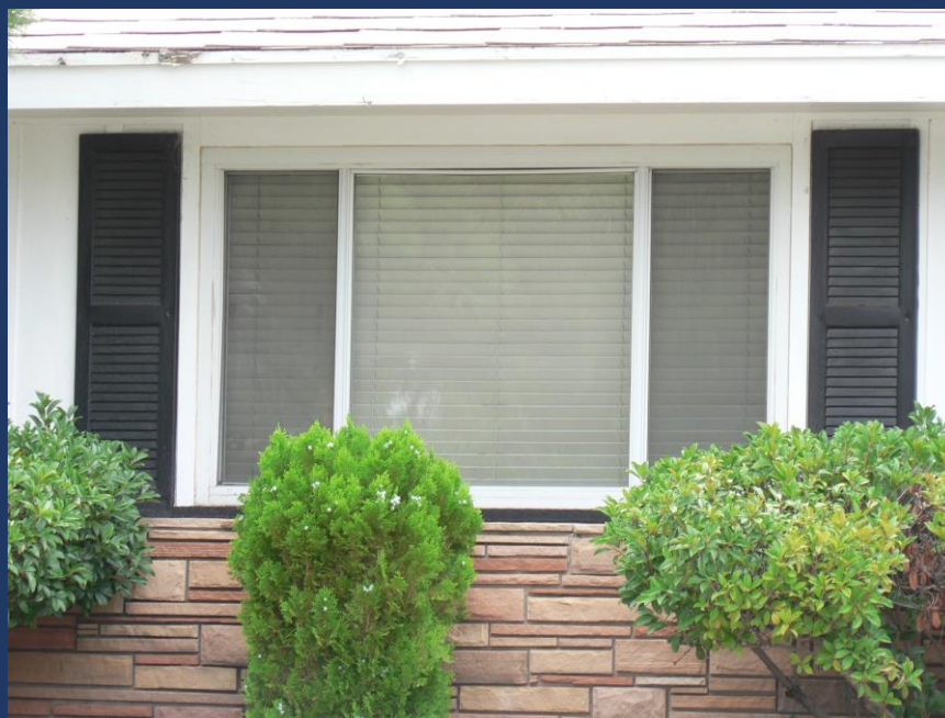
Ashlar Sandstone cladding
