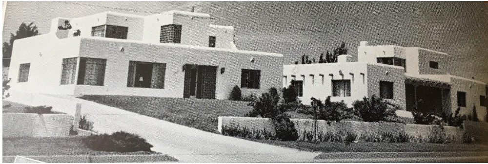
Two Streamline Moderne style homes constructed in 1947-48 on Ridgecrest Blvd. in Parkland Hills. Albuquerque Progress magazine photo.
