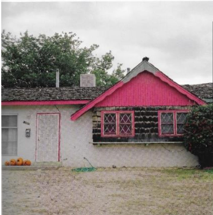
Cinderella (Storybook) Ranch homes in Princess Jeanne Park. (Top) Note the upturned gable ends, fanciful window trim, and original shake shingles on entryway. (Left) Home with original shake shingles on roof and siding of window box. Note original wood windows with cross-hatched mullions.
