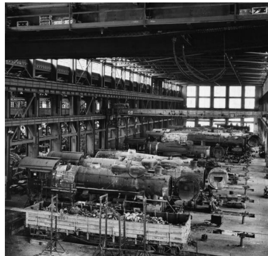
Locomotive shops at the AT&SF rail yards in the Barelás neighborhood.
