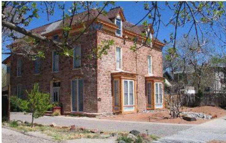
The Hesseldon House (1882) is an Italianate duplex in the Perea Addition.
