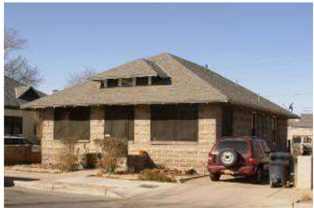
Hipped Box cottage on Eighth Street NW, ca. 1898-1902. The building material is cast stone.
